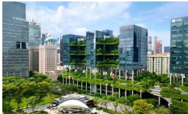
Investition in klimaneutrale Metropolen
